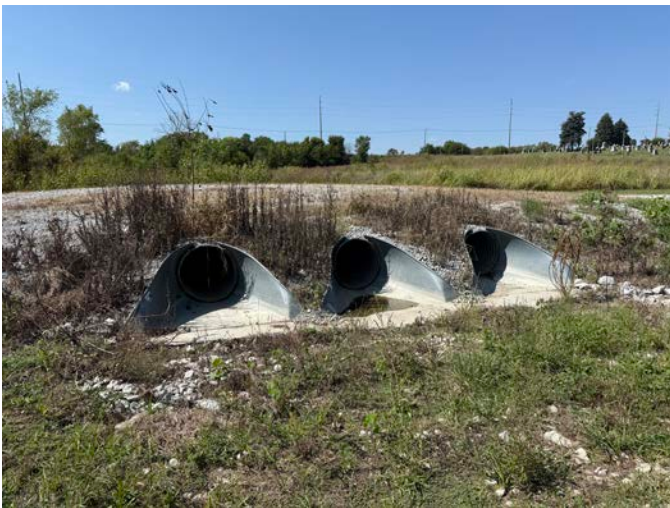
FIGURE 102 • EXISTING CULVERTS
