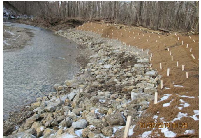
FIGURE 88 • BIOENGINEERED STREAM BANK
