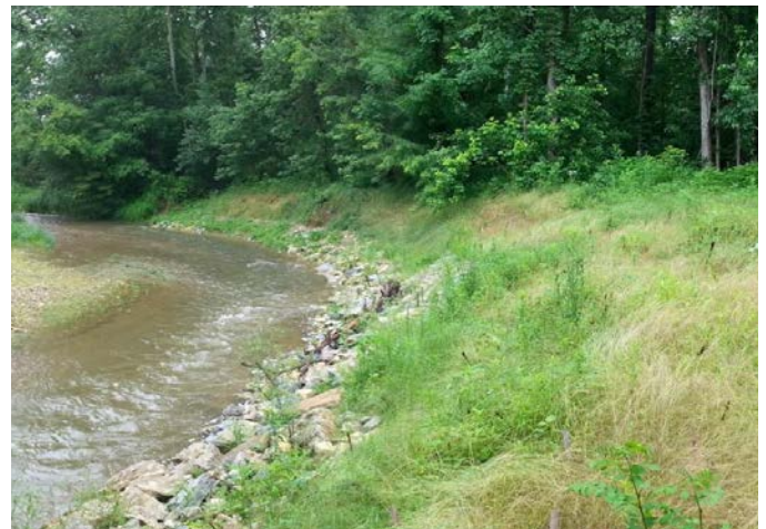
FIGURE 89 • RESTORED STREAM BANK
